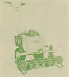
Reo Trimalawn 25" Deluxe mower power propelled, trimmer type mower that cuts a wide smooth 25" path. Eliminates hand trimming. Convenient handle controls, one for clutch and the other regulates speed. Full Floating cutting reel.
